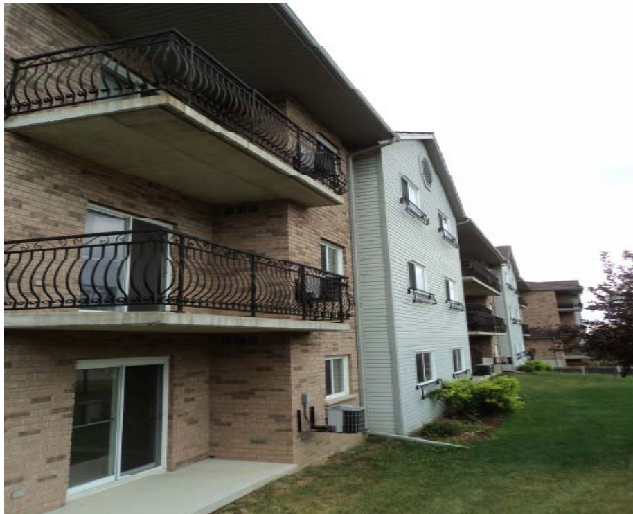
Photo 5 – Typical concrete balconies.
