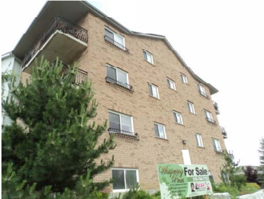
Photo 6 – View of north side of building.
