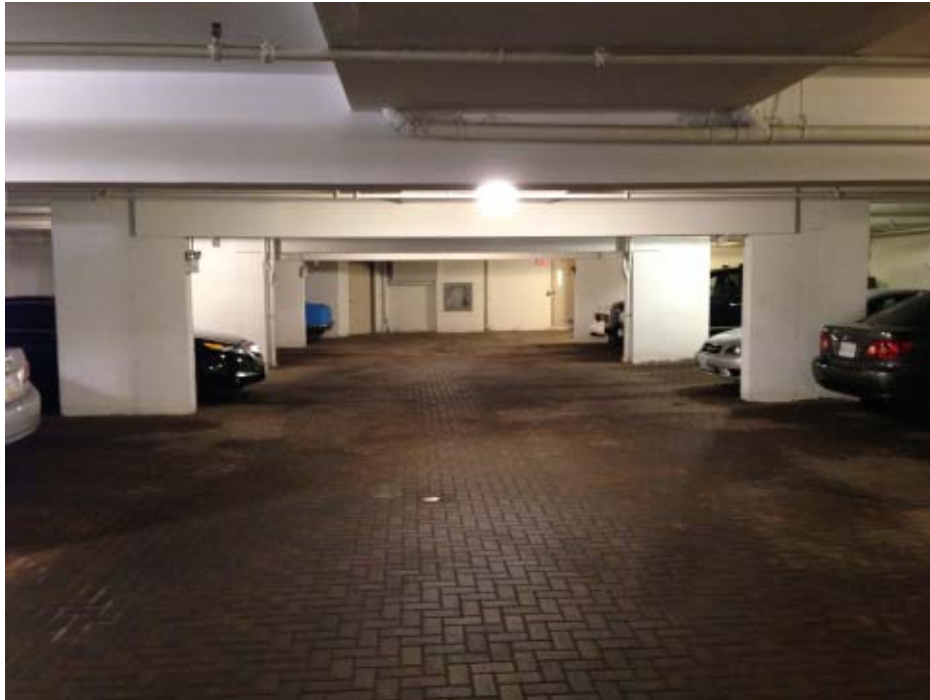
Photo 8 – Parking garage area with interlocking pavers.
