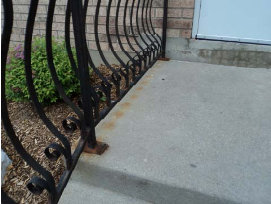
Photo 4 – South side stair railing
