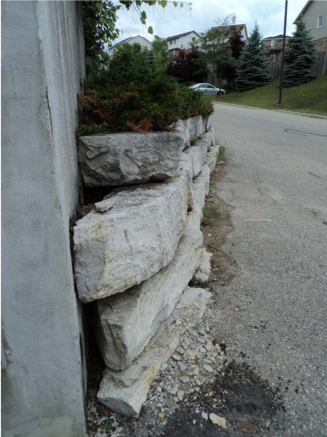
Photo 3 – Retaining wall west side of building by parking garage.
