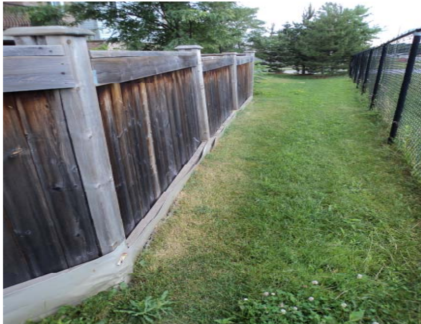
Photo 7 – Typical wood fence around patio area.
